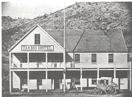
FIGURE 2-7. Idaho Hotel - July 1869 Block 4, Lots 78, 79, and 80. This building still exists today. See Figure 2-31.
